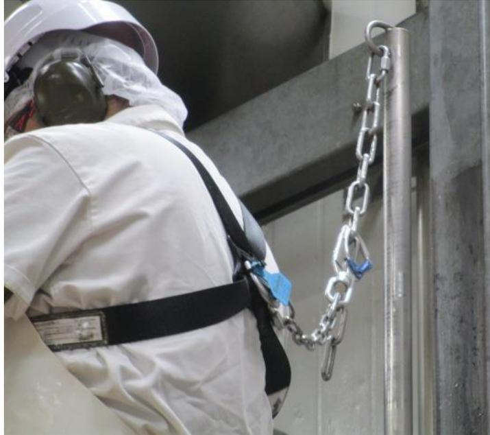
A fall arrest harness is intended to safely stop a worker falling an uncontrolled distance and reduce the impact of the fall. Only when a restraint system is not practicable, should a fall arrest harness be considered.
