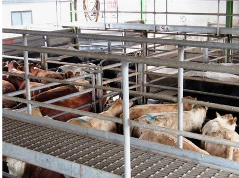
There should be railings along cat walks in yards. Consideration should be given for a gap at the bottom of the railing to allow for a person to climb out of the yard quickly.
